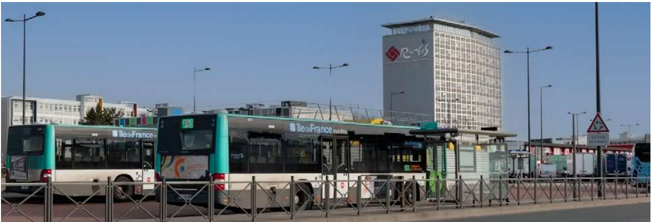
Bus station - Rungis International Market, France - Photo credit : Semmaris
