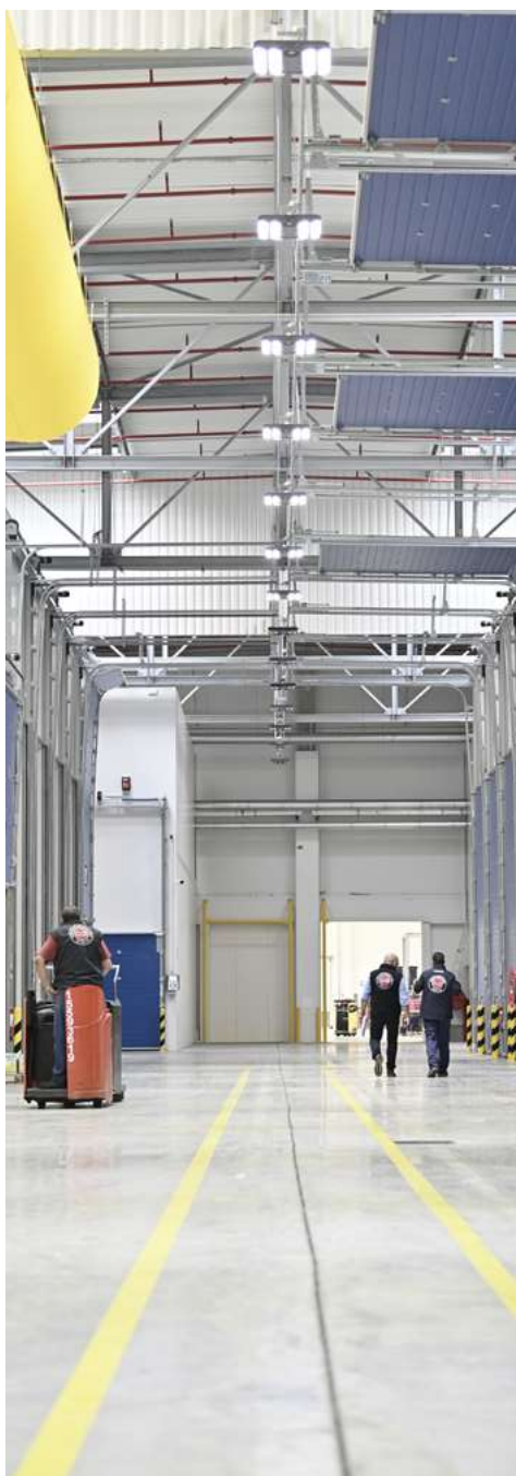
I1 Warehouse - SIIM, Rungis, France
